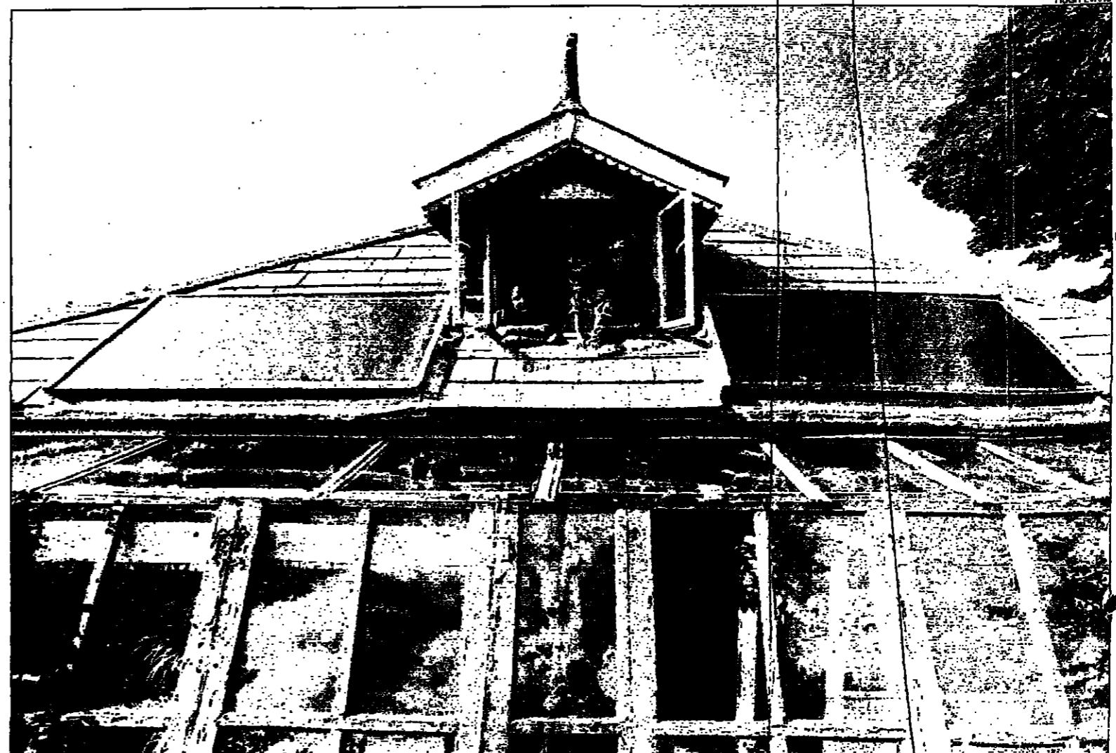
Two solar panels on the roof of the Smiths' house in Wales can heat a 250-litre cylinder of water, even when there is cloud cover
